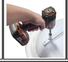
4. Using the supplied bolt & washers; attach the clawfeet to the bracket through the threaded hole on each end of the bracket.
